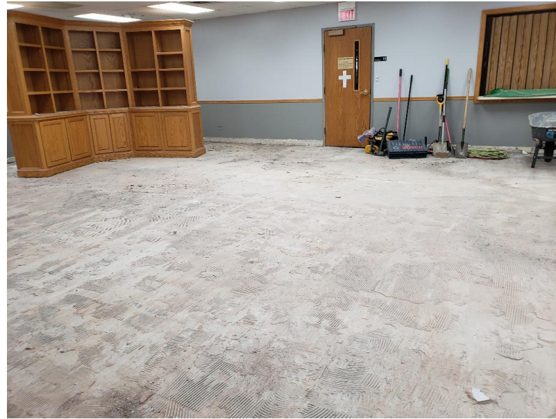
The fellowship hall during day 1. The noisy chiseling of the floor
